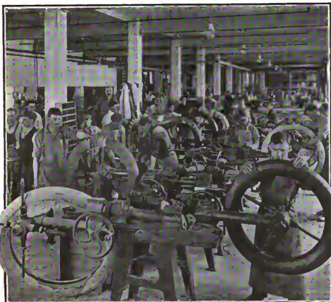
In the sundries room, showing arrangement of tire formers
